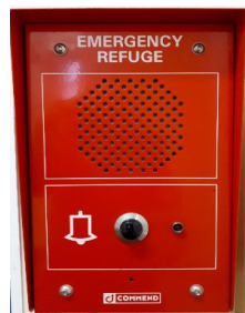
Commend refuge communications intercom
