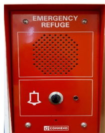
Commend refuge communications intercom
