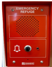
Commend refuge communications intercom
